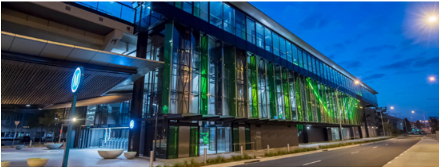
▲ Rouse Hill metro station
